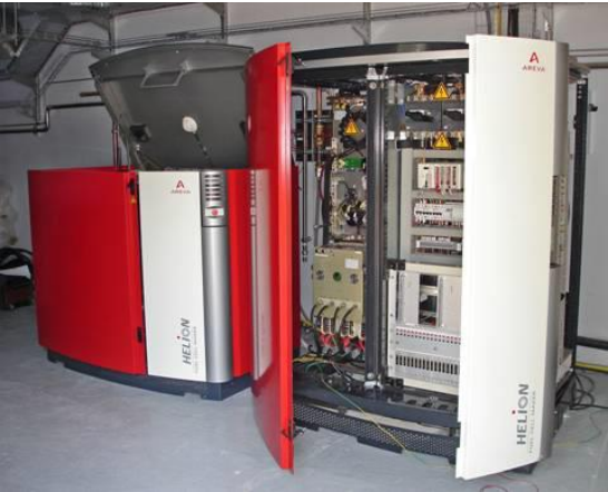
CEA SACLAY Back up system 30 kW, storage H2 200 bar, Range 8 h
