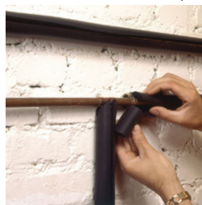
Illustration 3.9: Isolation des tuyaux
